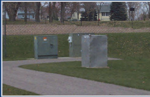
Wellhead pitless adapter with protective covering
