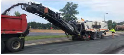
Removal of the existing street surface by milling
