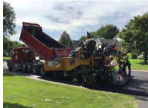
Installation of new asphalt surface
