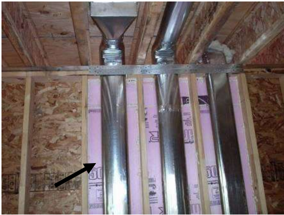
7. 1 1/2 rigid foam insulation used behind heat runs in exterior walls.
